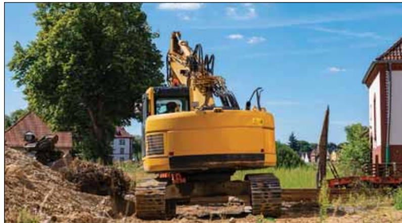
An excavator maneuvers past a tree during construction on a property.
