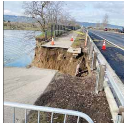
A segment of the trail pathway adjacent to Stanley Boulevard collapsed last weekend.
