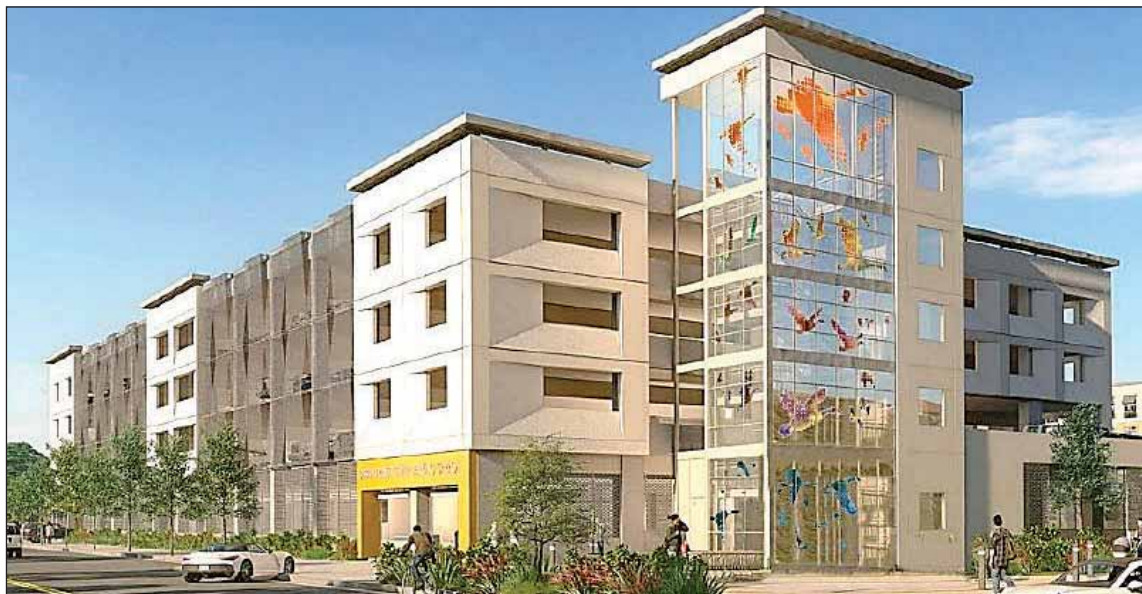
Rendering shows design concept for the new Dublin Transit Center parking garage now under construction.
