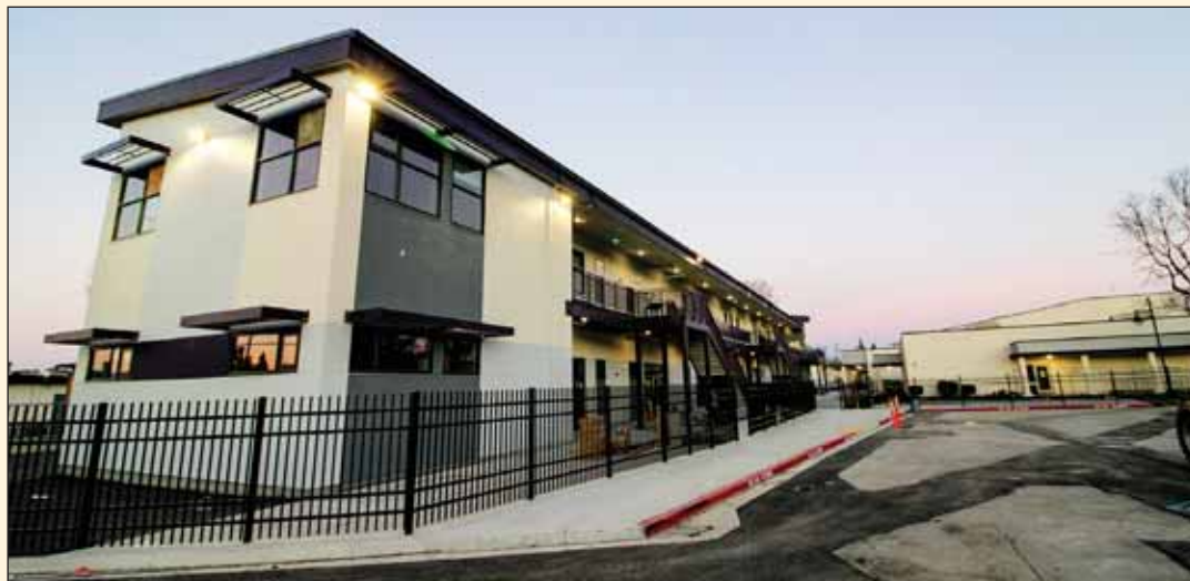
The new classroom building at Amador Valley High School, a project funded by Measure I1, has been wrapped up this summer.
