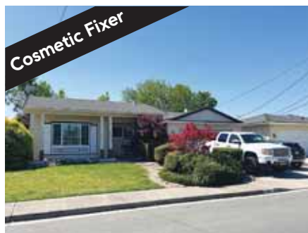
6664 Maple Drive, Dublin 3BD, 2BA, 1446sf SFR Newer Roof, Windows, Furnace & W.H. Listed @ $1,188,000 Call Steve @ 925.580.8011 to Submit An Offer Prior To Market
