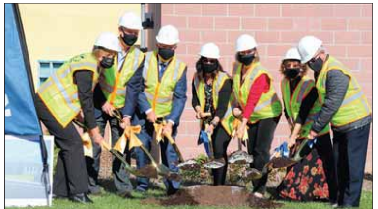
School and district officials ceremonially break ground on the first phase of the Hart Middle School science building project.
