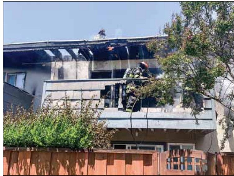
Crews work to control the fire scene in a Livermore apartment complex on Tuesday afternoon.
