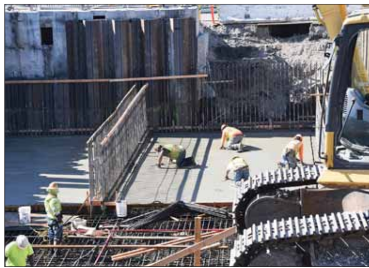
Construction workers smooth out freshly poured concrete for the base of the two new primary sedimentation tanks.
