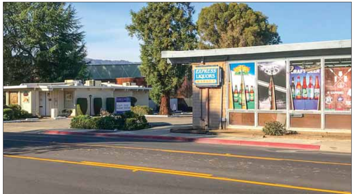
The city has closed escrow on its purchase of this downtown commercial property at 4363 and 4377 First St., which includes these two buildings. Tenants were offered relocation compensation.
