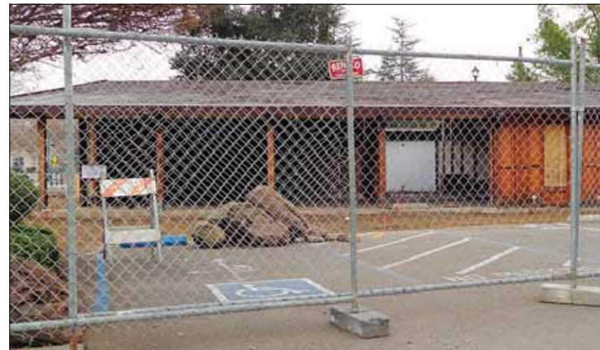
Once home to the former Panda and Joy China restaurants, this building at 30 W. Angela Sidetrack, a family-style restaurant and bar that will open this summer.
