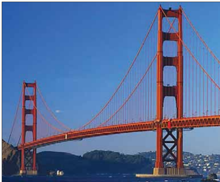
Golden Gate Bridge
