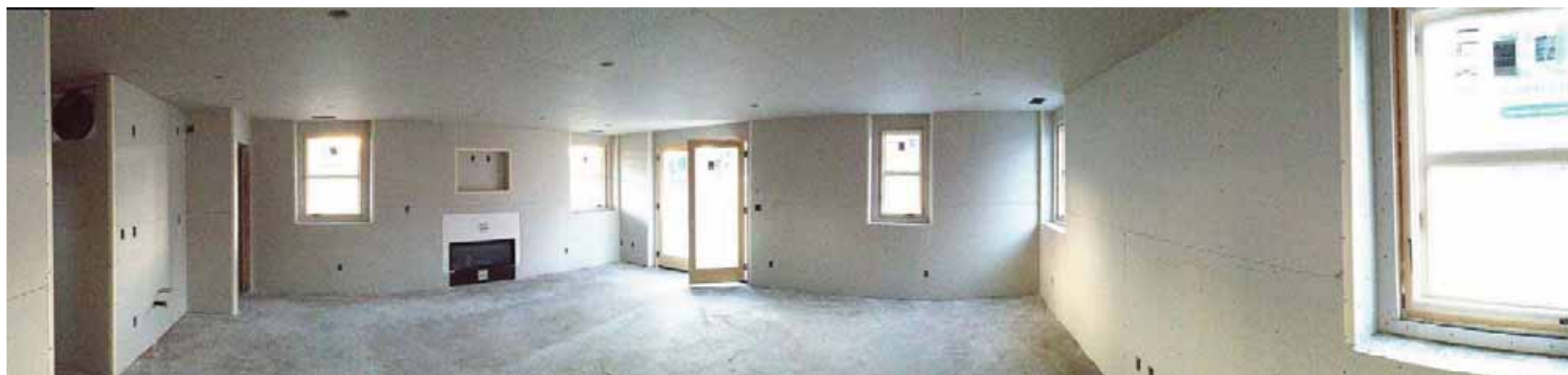
A panorama view of part of the basement during the renovations.
