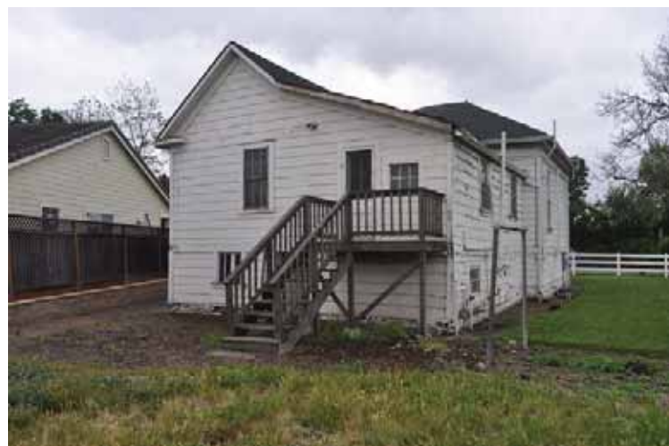
The remodeling and restoration got underway when the Machis tore down this 1940s addition to the house (shown in foreground).
