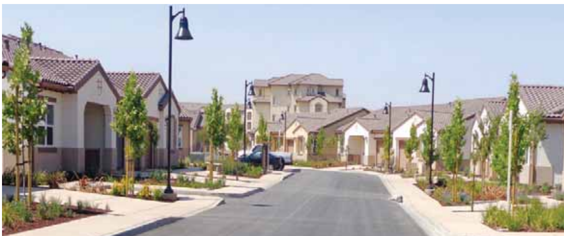
Street scene at Stoneridge Creek shows mix of independent living homes with four story apartment building still under construction. So far, 280 homes have been reserved with 134 in the current construction phase still available.
