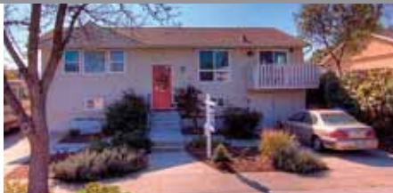
CAMPBELL Open SAT/SUN 1 - 4 3890 BUCKNALL ROAD NICELY UPDATED HOME! $749,800 3 BR 2 BA Kit w/Quartz counters & new appl.In-Law quarters.New dual pane windows & carpet.RV parking 925.847.2200
