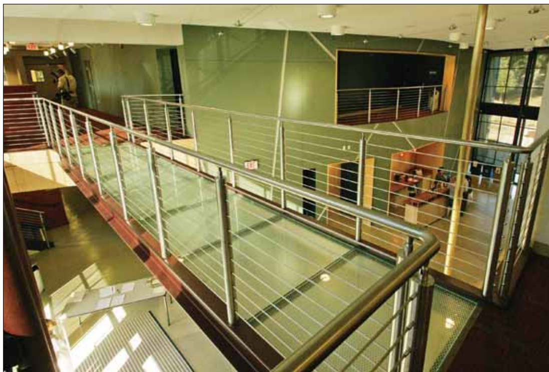
A steel walkway with a see-through bottom connects art studios, classrooms and exhibit area on the second floor of new Firehouse Arts Center.
