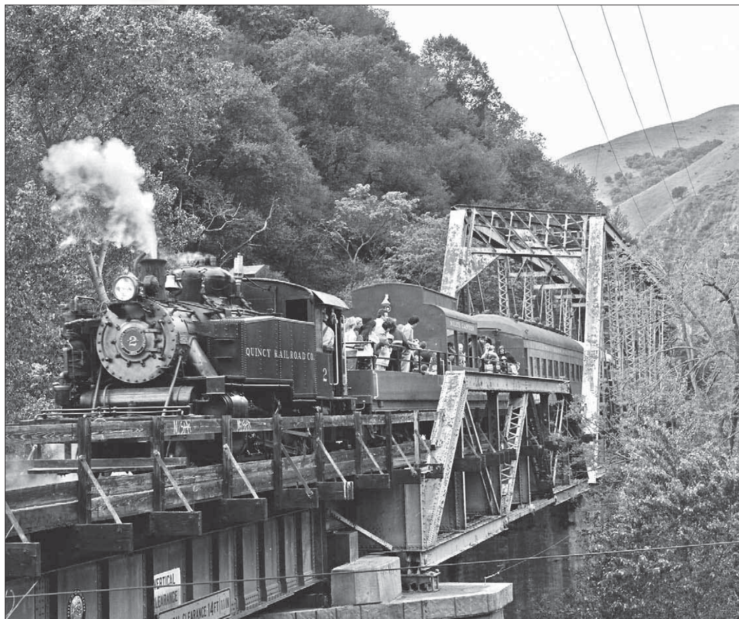
An excursion train passes through the Farwell Bridge, one of two bridges through Niles Canyon. The 1896 truss is still supported by stone piers, which 2002. The same bridge, originally constructed in 1865-66, is also seen in the postcard in the top right of the next page.
