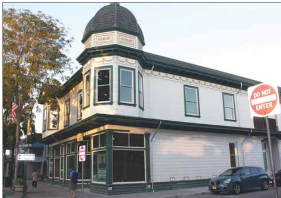
After the Planning Commission's denial of an appeal for an ATM to be installed on the side of the historic Kolln Hardware building, the machine will be allowed for Comerica Bank, which will occupy the first floor.
