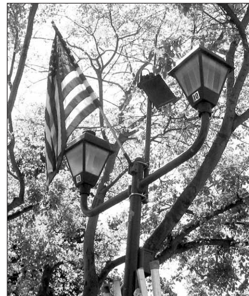
Access points have been installed on lamp posts.
