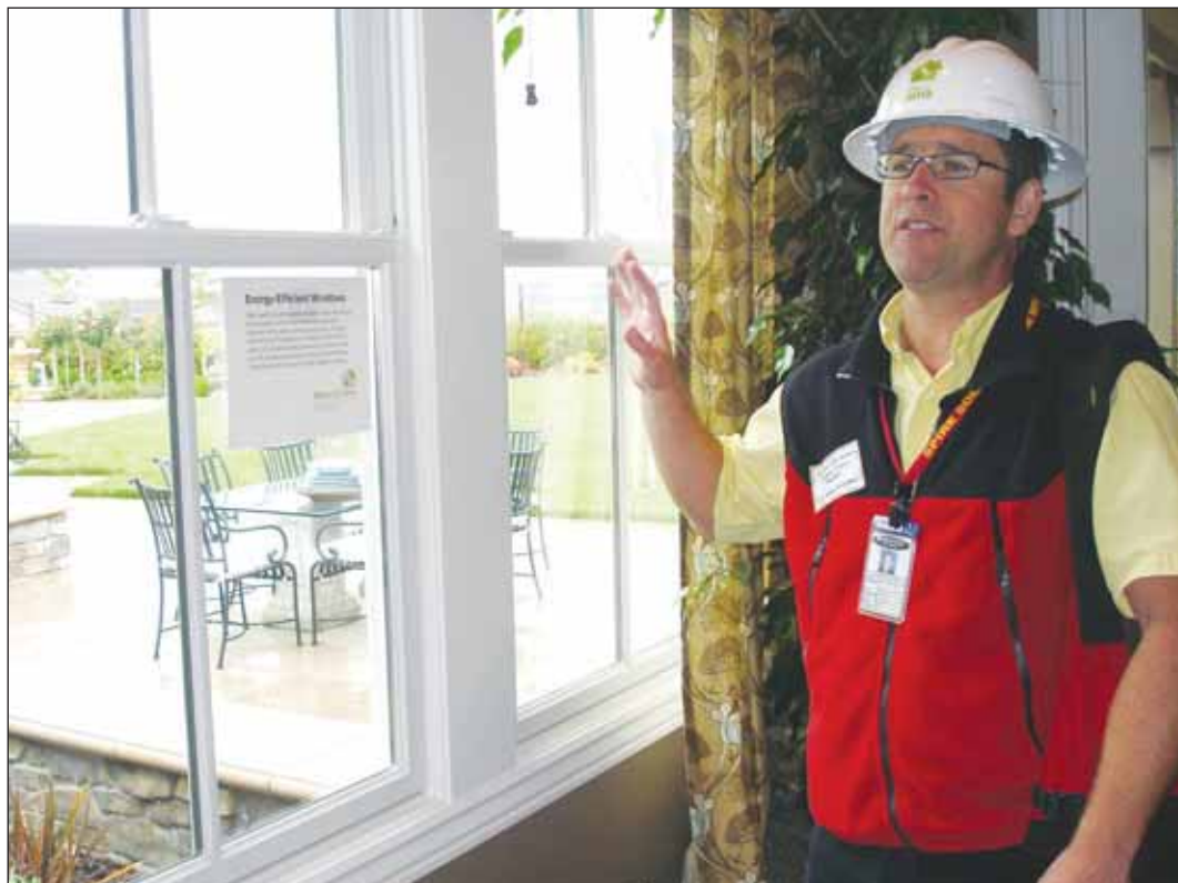
Kevin Gilleran rates the level of "green" features used in a home and calculates points earned. Double-paned, low-E coating windows as seen in a home in the Avignon by Centex development off Vineyard Avenue reflect heat, saving the homeowner on his or her electricity bill.
