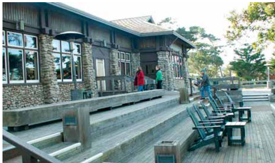
The Phoebe Apperson Hearst Social Hall, paid for and named after Pleasanton's most famous resident, was built in 1913. Architect Julia Morgan used poured-in-place concrete for the foundations and exterior walls, creating an informal lodge feeling by concealing the concrete beneath a wood-and-stone exterior. All guests register here.
