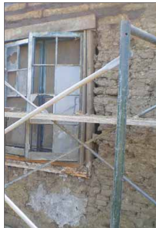
In order to maintain the historical integrity, much of the renovation, including brick making and plastering, was done by hand.
