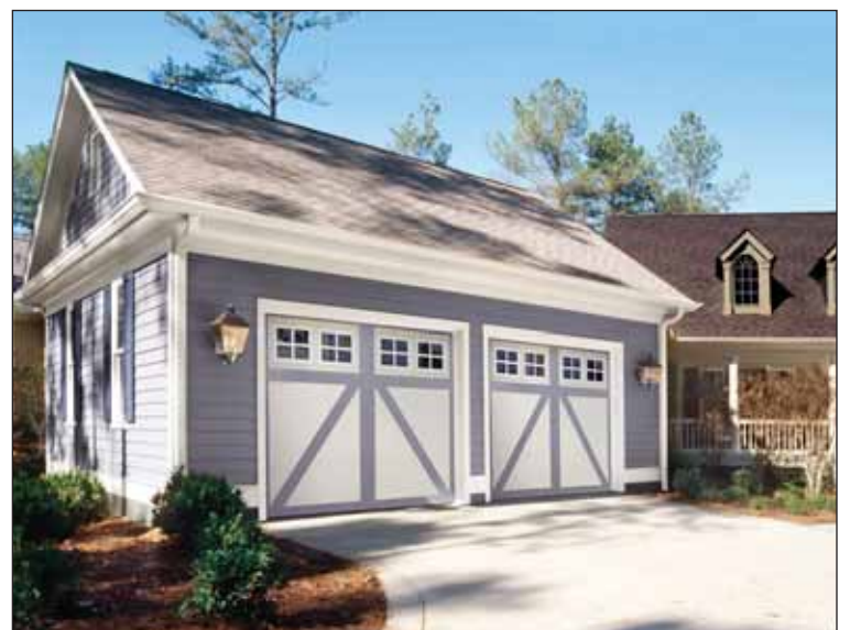
To green the garage, consider replacing the garage door with one made from 100 percent recycled wood fibers.
