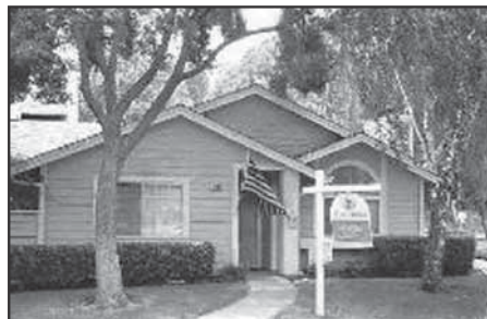
Pleasanton – Charming, single story end unit with 2 bedrooms, 2 baths, 1173 square feet of living space, hardwood floors, newer carpet and paint, newer appliances, refrigerator and washer stay. Lots of storage space, 2 patios, and a wood burning fireplace. Clean as can be, this is a must see, located next to park like greenbelt! 7303 Stonedale Drive $499,900
