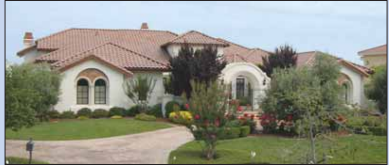
1297 Via Di Salerno - Wonderful custom home back on the market with 200k price reduction. $2,795,000. 6300 sq. ft. home on the golf course with dramatic views of Diablo setting sun.
