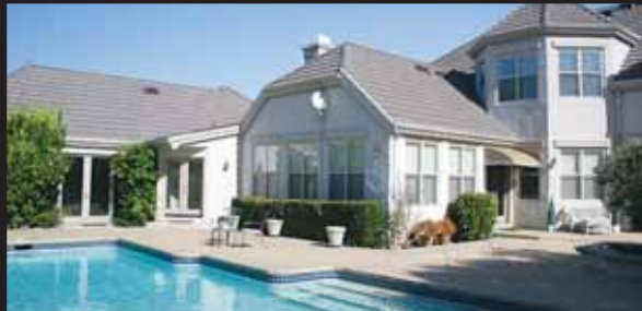
Pleasanton – Beautiful CUSTOM Home in Ruby Hill with a Courtyard Area-PorteCochere. The OUTDOOR area features POOL, SPA, BBQ, Fireplace and Views. The First Floor has a huge Kitchen Nook, Family Room, Guest Suite, Office and a Bonus Room. All of this and Privacy too! 3019 E. Ruby Hill Drive $2,199,000
