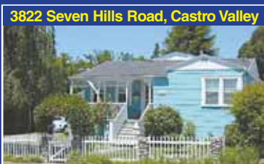
3822 Seven Hills Road, Castro Valley
